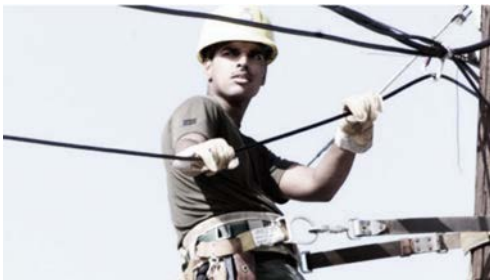
Figure A-20 Line Technician
